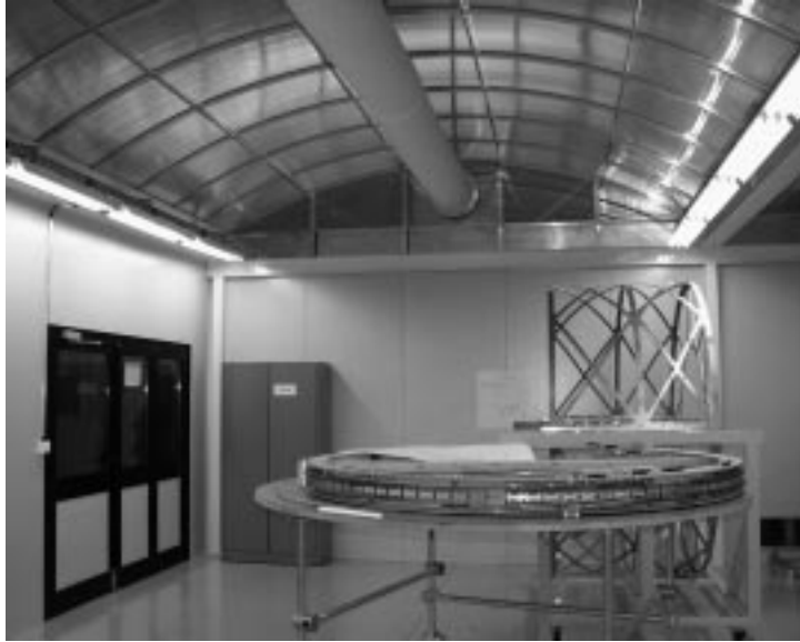
Figure 2: Flexible ventilation duct in Bldg 154.
